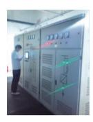
Regenerative braking energy absorption inverter (35kV feed)
